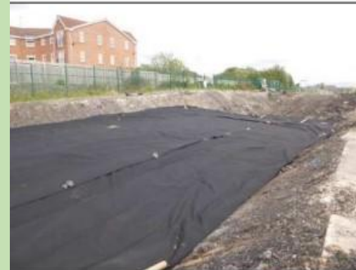
Image 3 – Sealing of the cell prior to clean cover being placed
