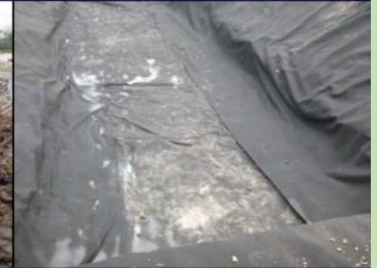
Image 2 – Lining the cell with CuTex
